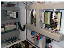
The M0200 continuously reads engine speed, oil pressure and cooling water temperature from the ECM of the engine. Readings are transferred to the M2000 from the discreet contact outputs. The M0200 supports the cable check function of the M2000.
